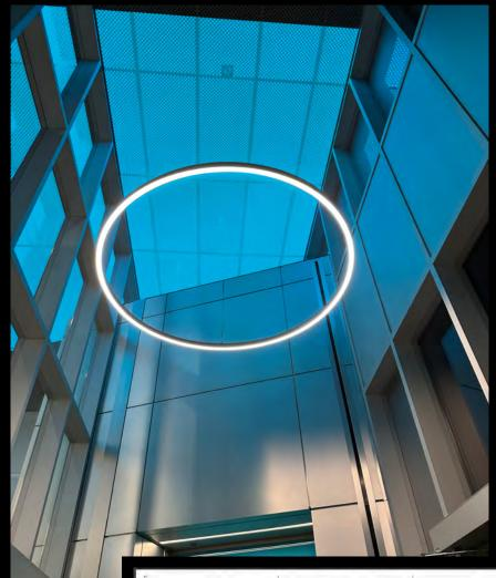
Fitting these backlit LED panels into the pre-existing structure required the kind of attention to detail, coordination and support that EOS is well known for. The process began with measurements & approved drawings, and followed with a test run of initial LightPanels for proper fit, only to follow with the full production run of 90 overhead RGBW luminaires.
