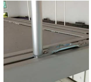
Suspended CLOUD MEDIA FRAME by rigid poles
